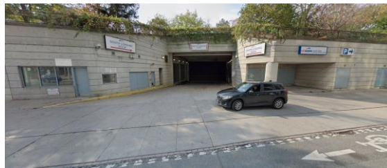
Entrance to Loading Dock, South Building
