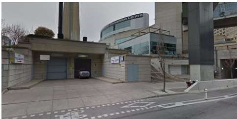
Entrance to Truck Elevator, South Building
