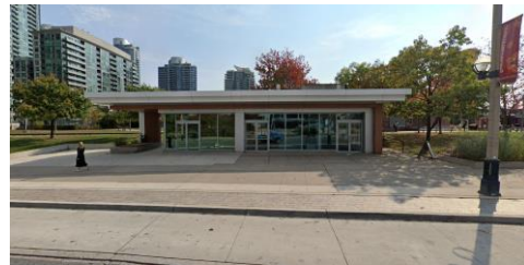
Bremner Service Elevator, South Building
